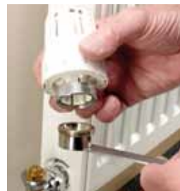
2. The thermal ring is screwed into the threaded adaptor at the base of the tool. This compresses the clips on the TRV head and allows the ring to pop off. The ring becomes more difficult to turn as the compression increases and it is sometimes necessary to use grips to increase leverage.
