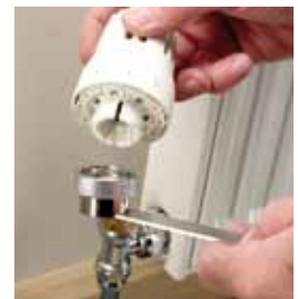
3. The head can then be pulled free of the thermal ring, leaving the ring attached to the tool.
