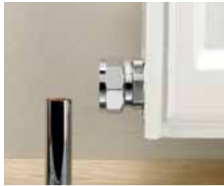
2. The tailpiece is screwed by hand into the radiator.
