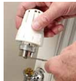
2. The thermal ring is screwed into the threaded adaptor at the base of the tool. This compresses the clips on the TRV head and allows the ring to pop off. The ring becomes more difficult to turn as the compression increases and it is sometimes necessary to use grips to increase leverage.
