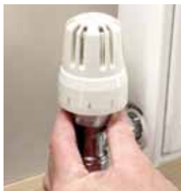
1. The TRV head is removed from the valve body by unscrewing the thermal ring.
