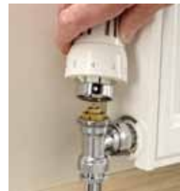
6. The secure thermal head can then be re-attached to the valve body, tightening by hand.
