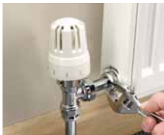
2. The tailpiece is tightened into the radiator.
