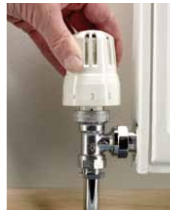
4. The head is pushed down, locking it into place.
