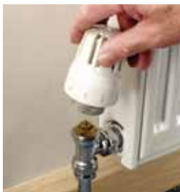
1. The TRV head is removed from the valve body by unscrewing the thermal ring.
