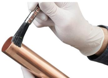
**2.** Insert the tube into the fitting until it reaches the tube stop, using a twisting action to ensure the spread of flux. Ensure the tubes are correctly lined up and adequately supported – otherwise distortion or cracking may occur when at brazing temperature.
